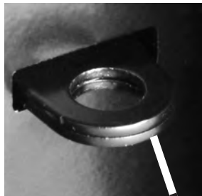
Double-thickness padlock loop with 10mm diameter aperture
